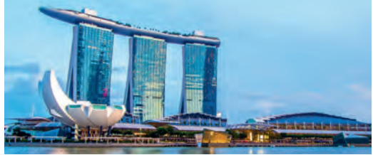
SPP project: Marina Bay Sands - Singapore
